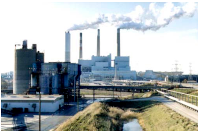
Figure 1-1. Flue gas desulfurization (FGD) product is created by a scrubber that removes sulfur dioxide ( \text{SO}_2 ) from the flue gas stream when energy sources containing high concentrations of sulfur are burned. (Norton and Rhoton, 2007.)
